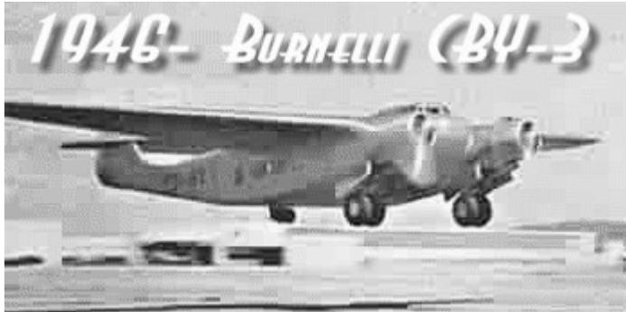
**Vince Burnelli's 1946 CBY-3** had a 20'x20'x6' cargo-passenger bay, could carry a ton more than a DC-3 with the same engines, and got 40% of its lift from the airfoil-shaped fuselage.
